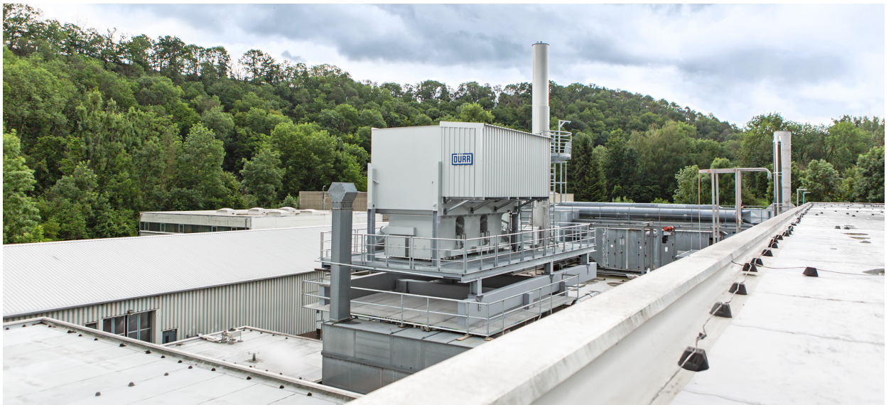
Picture 2: Compact and pre-installed RTO Oxi.X RK
